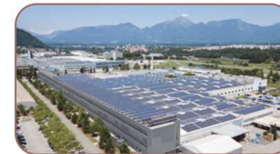
3.38 MW Iskra PV systems combined
