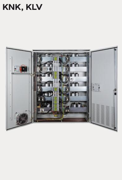
Power factor correction (PFC) aims to improve power factor, and therefore power quality. It reduces the load on the electrical distribution system, increases energy efficiency and reduces electricity costs. It also decreases the likelihood of instability and failure of equipment.
